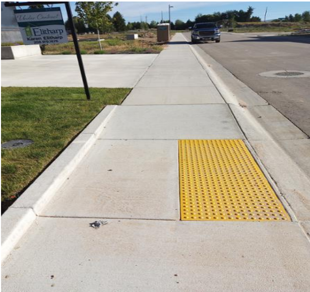
Photo to show the front sidewalk.
