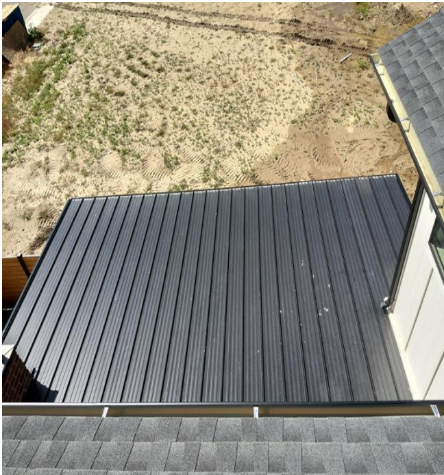
Photo of the porch roof. Example of roof #2.
