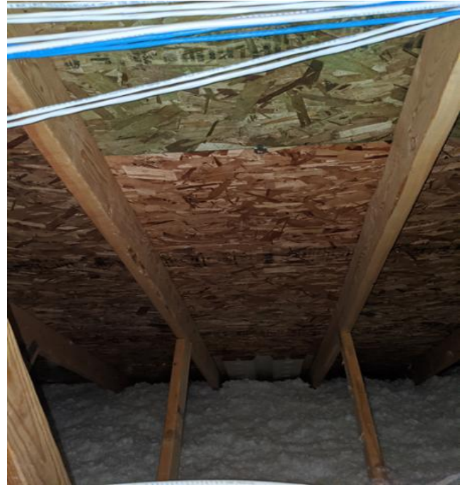
Example of the OSB roof sheathing.
