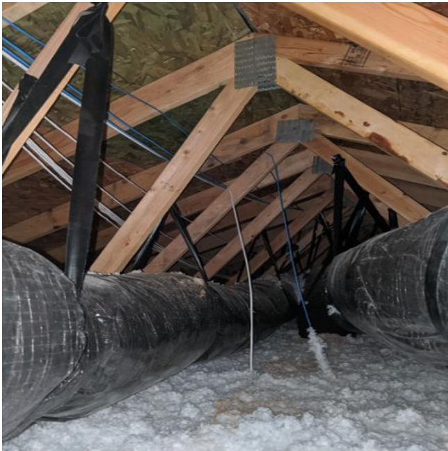
Photo to show example of the trusses in the attic.
