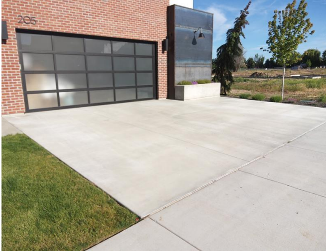
View of the concrete driveway.
