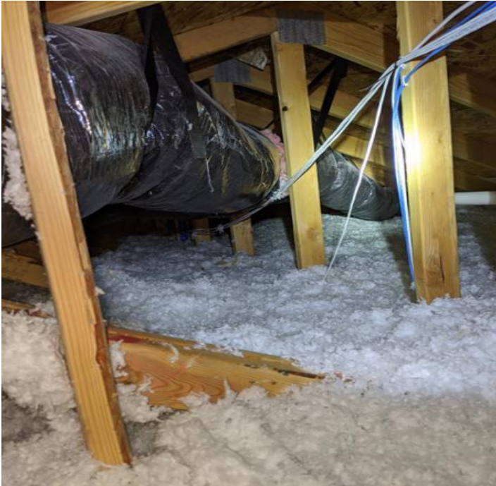
Another view of the attic.
