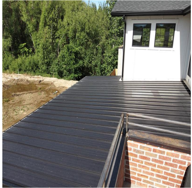
Example of the satisfactory condition of roof #2.
