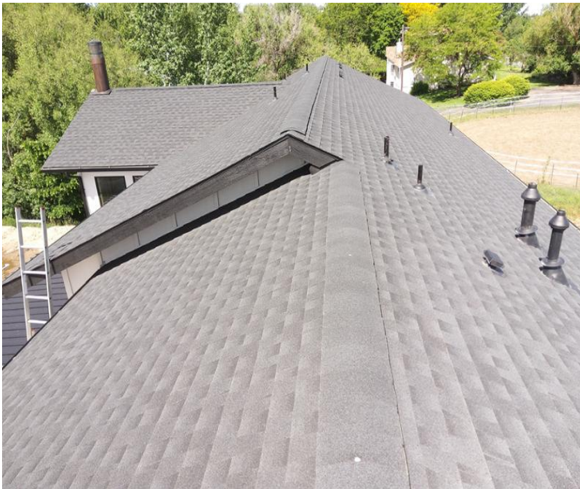
General view of roof #1.
