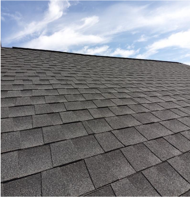
Photo to show example of the satisfactory conditions of the roof #1.
