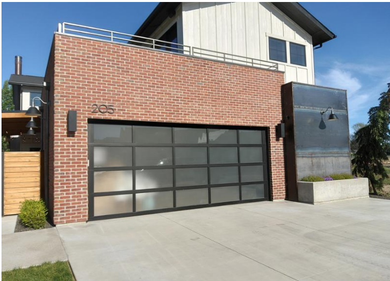
Photo to show the garage type.
