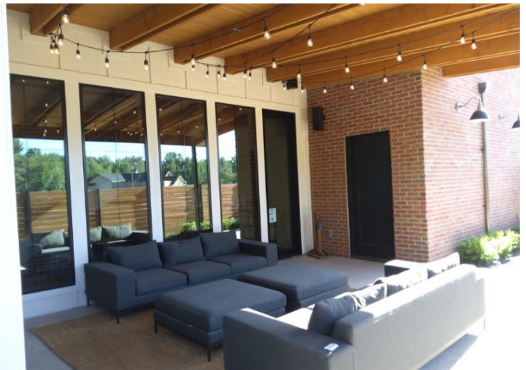
General view of the porch.
