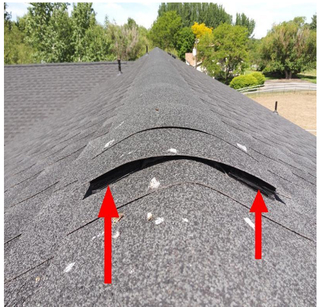
Arrows to indicate examples of the ridge vents.
