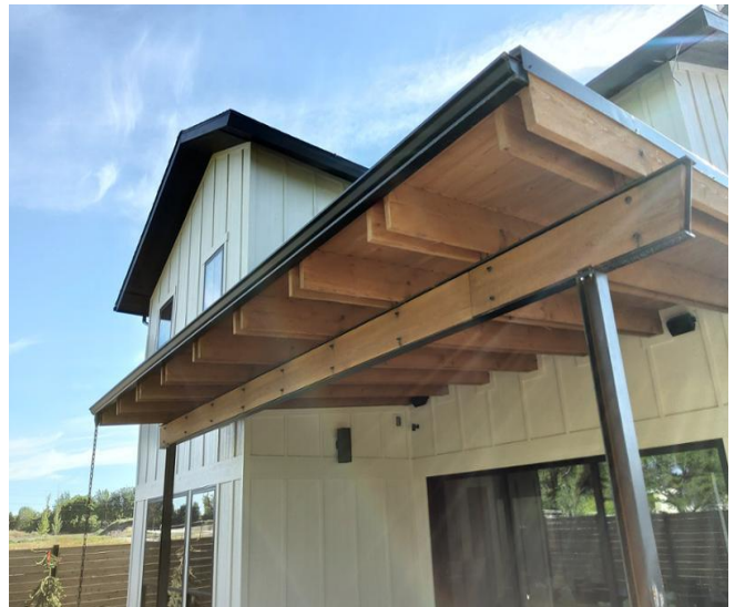
Photo to show the back-patio roof covering.
