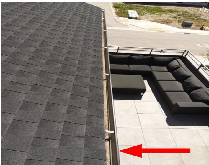
Photo of the gutters at the balcony roof.
