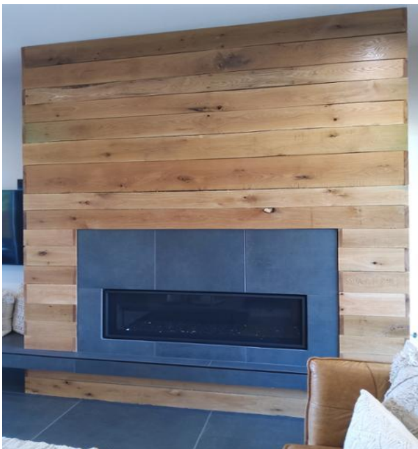
General view of the gas fireplace.
