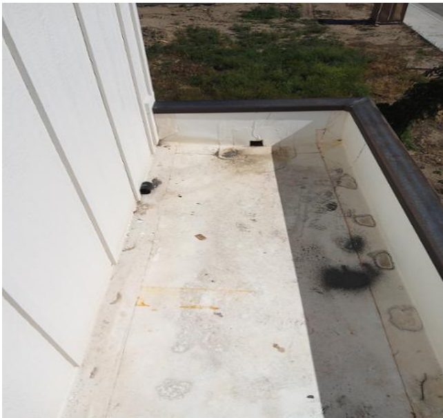
Example of roof #3.
