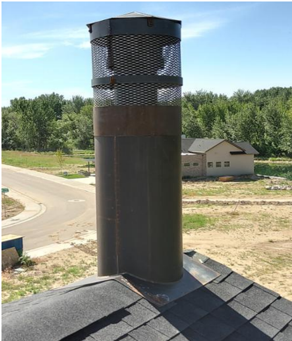
General view of the chimney.
