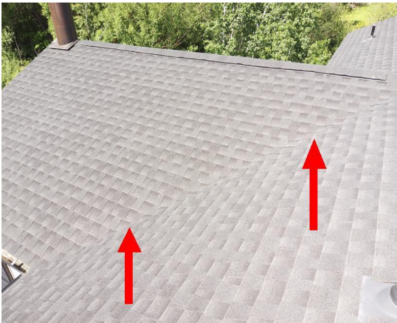
Photo to show example of the asphalt valleys.
