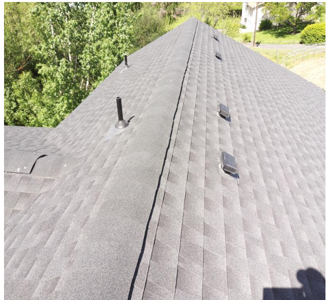
Example of roof #1.
