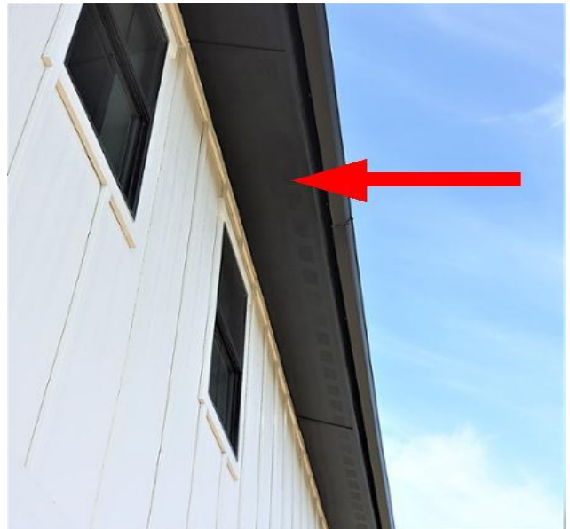
Arrow to indicate example of the soffit.
