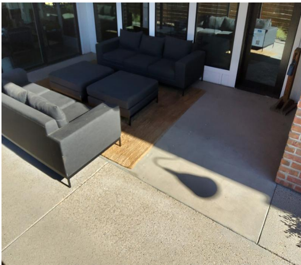
Photo to show the concrete floor.
