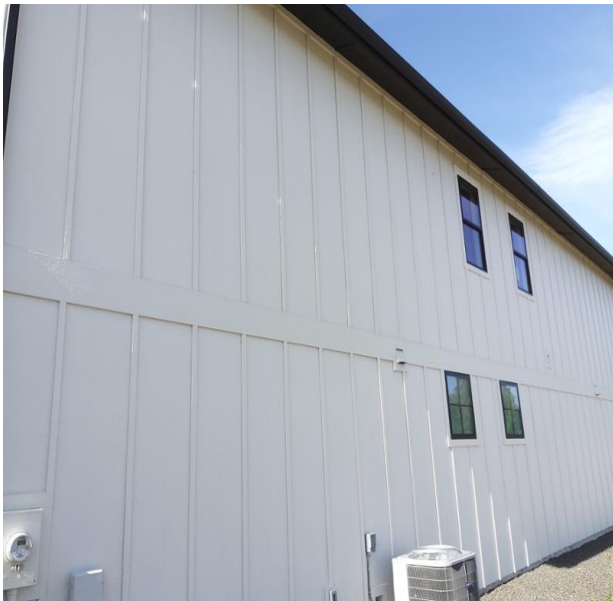
Example of the siding at the north side of the house.
