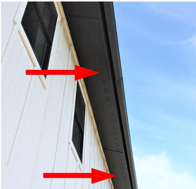
Arrow to indicate example of the soffit vents.
